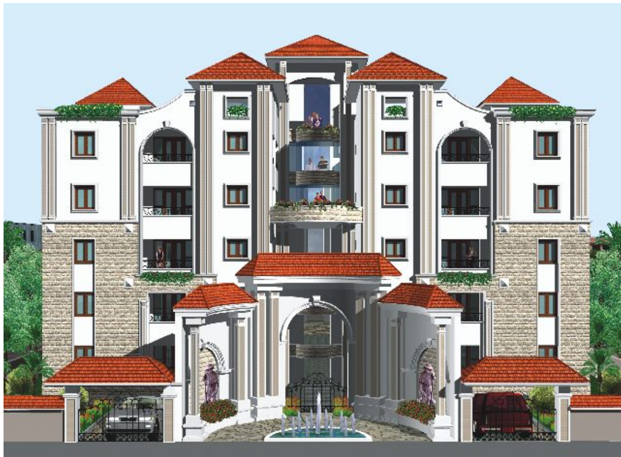
▲ ACE Monte Carlo at Kothaguda (Completed Project)
